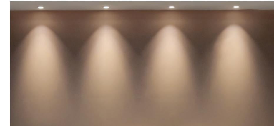
A few HOLLOWs close to the surface are a great idea to emphasise it. The closer to the wall a luminaire will be mounted, the more prominent the light beam will be.
